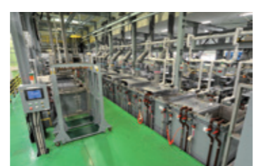
Chemical processing line
